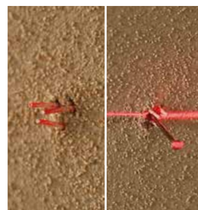
Elastic “stubs” to permanently ensure surveyed measurements are securely marked until after plastering work.
