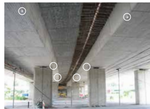
Observation of bridges
