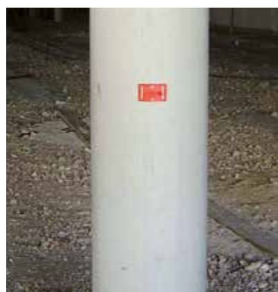
RS21r* fixed to a column. The protrusion is cut in 4 - 5 times with a carpet knife.
