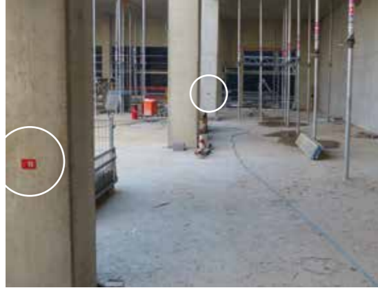
RS30r in industrial construction: documentation of heights and axes in one product.
